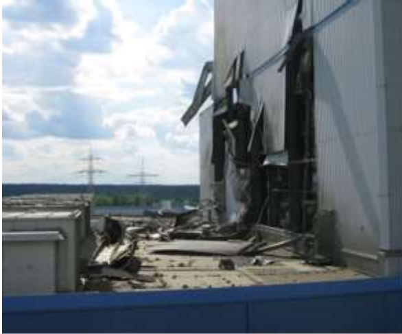
Damage at facade boiler house unit 5
