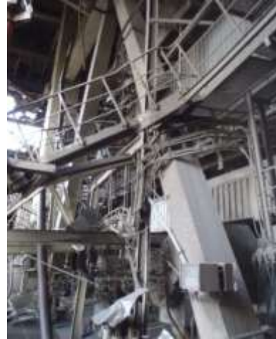
Damages at steel structure
