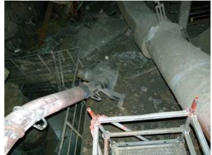
Upper part of pump casing ripped off
